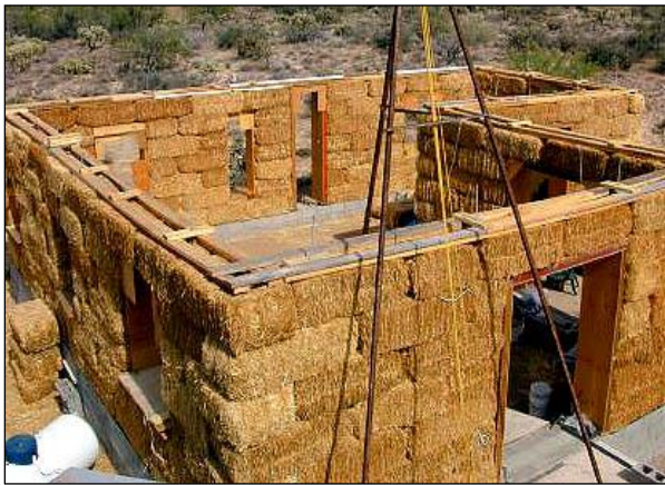
Figure 6: Using the wood pars to prevent bales sliding.
