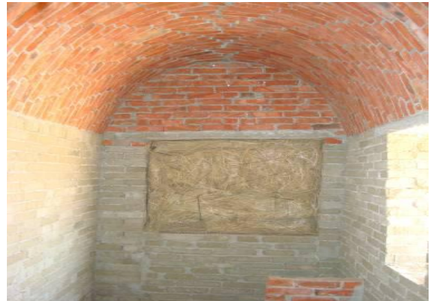
Figure 11: The vault by R-brick and red- brick
