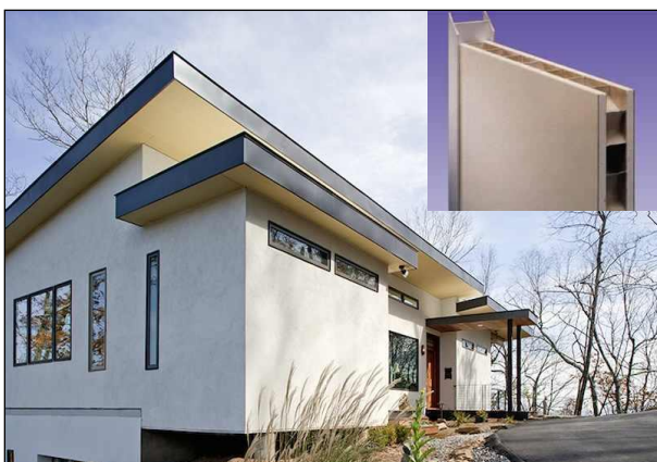
Figure 8: A house by the rice straw compact panels.
