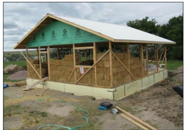
Figure 7: Non-load bearing structure
