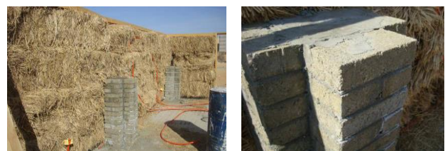
Figure 12: The 6 corner made of R-bricks
